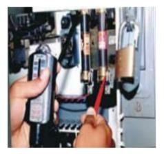
Worker was performing testing on the circuit without PPE. What should have been done before the cover was removed?
